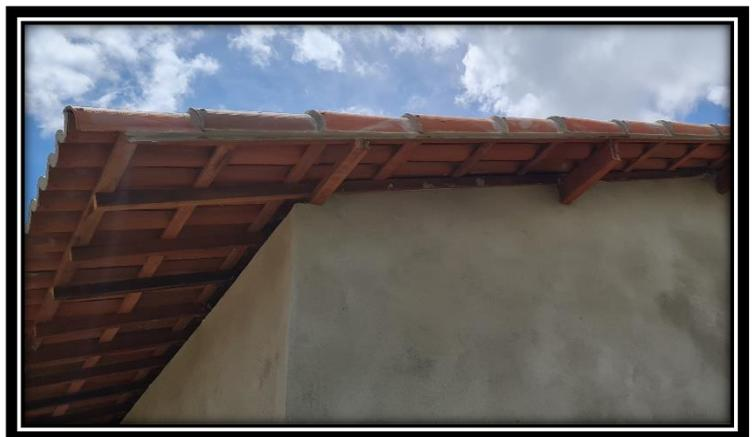
06.02 - TELHAMENTO COM TELHA CERÂMICA CAPA-CANAL, TIPO COLONIAL, COM ATÉ 2 ÁGUAS, INCLUSO TRANSPORTE VERTICAL. AF\_07/2019
